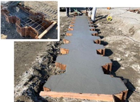
Fig. 3. RC Connection
