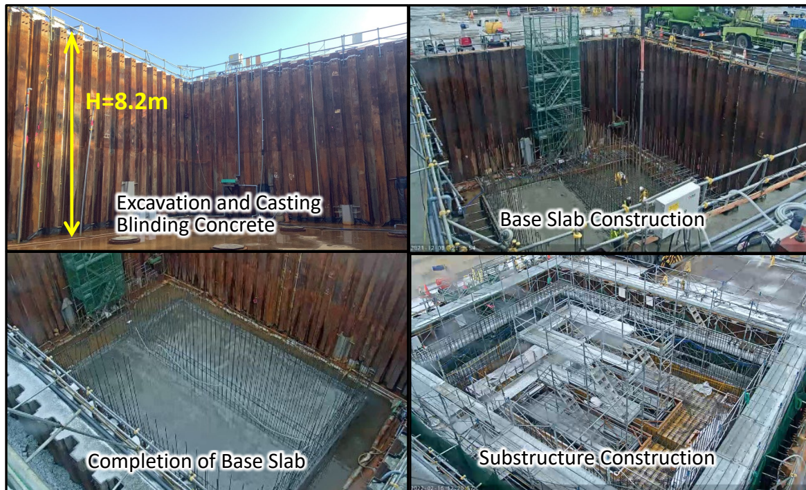
Fig. 6. Excavation and Construction of Substructure
