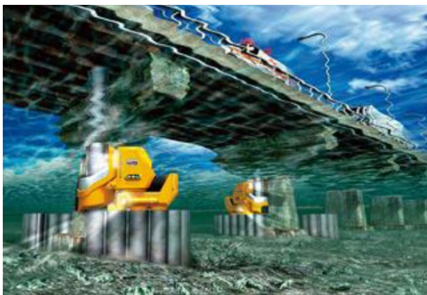
Fig. 2. (a) Press-in piling solution for scour
