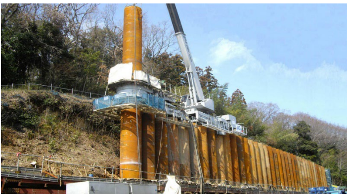
Fig. 4. (a) Implementation of an embedded retaining wall
