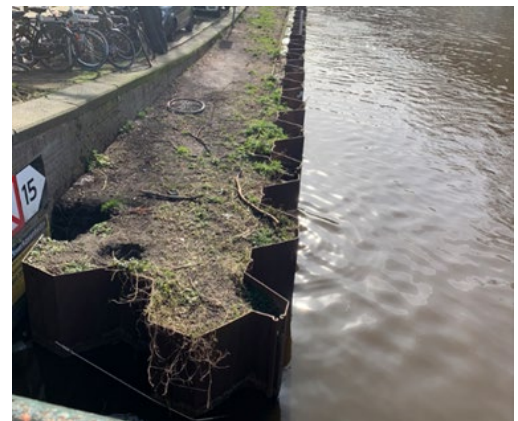
Fig. 2. Remedial works installed for temporary stabilization
