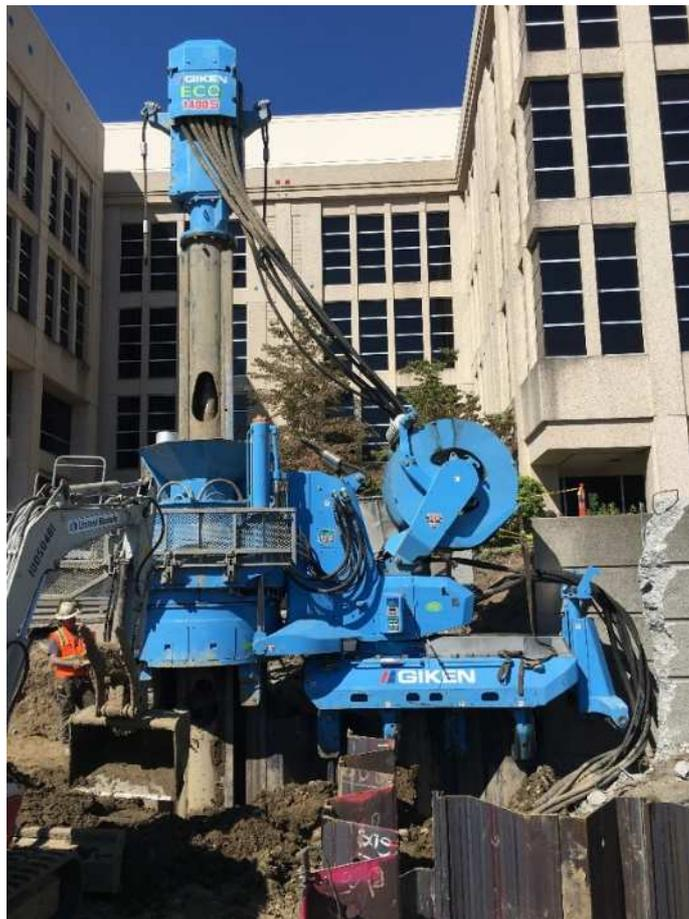
Fig. 3. Press-in piling with auger attachment
