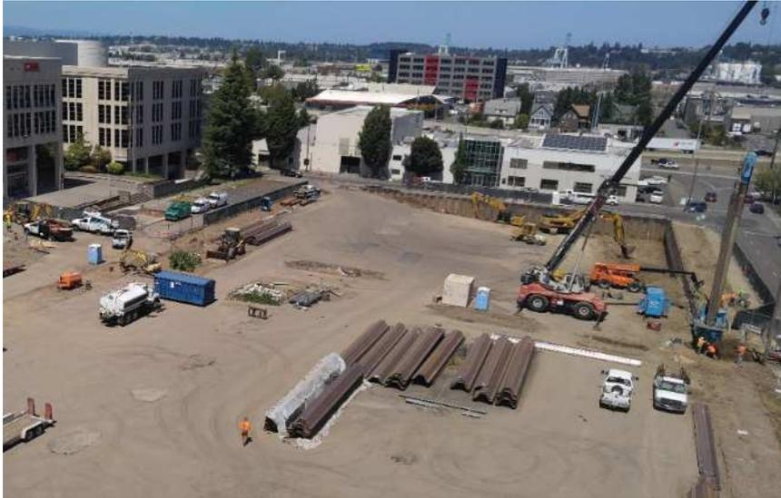
**Fig. 4. Press-in piling (far right) followed by excavation**
