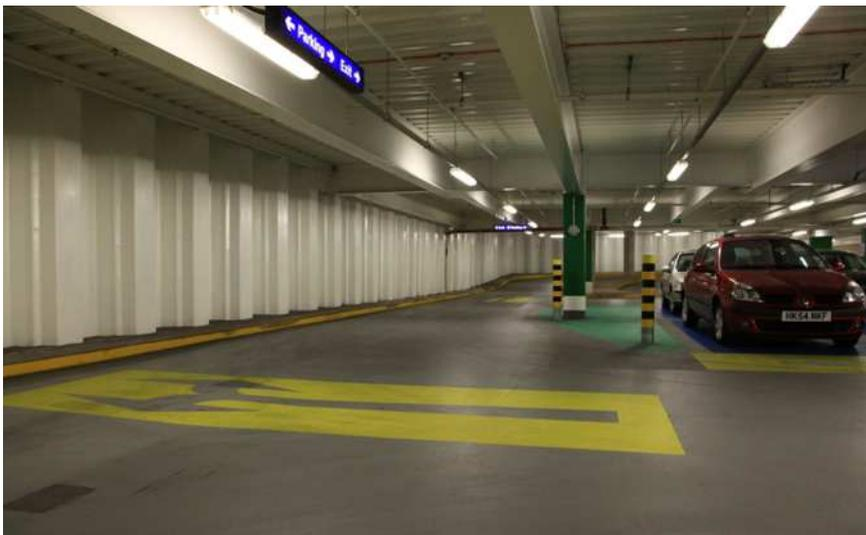
**Fig. 5. Example of completed basement with sheet piles (different project)**
