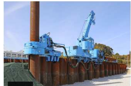
Fig. 3 Overview of Combi-Gyro Method
