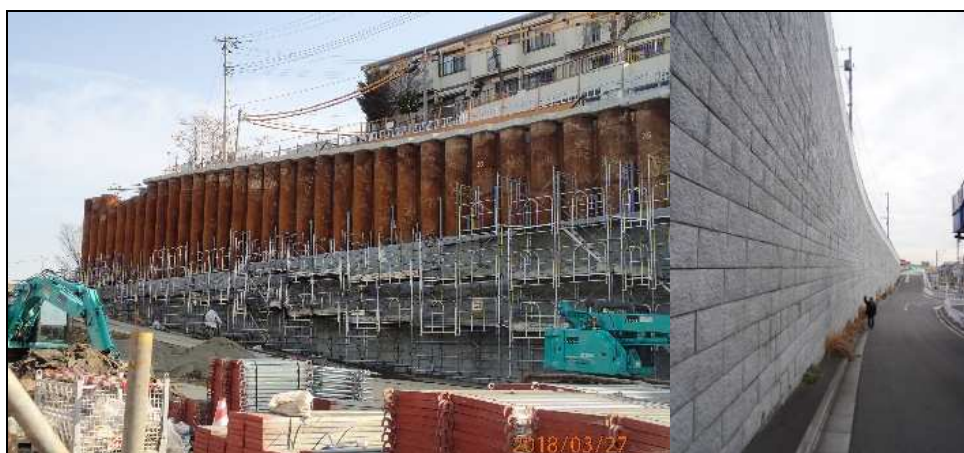
Figure. Baba Interchange, Yokohama Ring Highway. Left: retaining wall construction by Gyropiper, right: completed wall with Dr. Takemura
