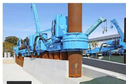
Fig. 2 Overview of Gyropress Method
