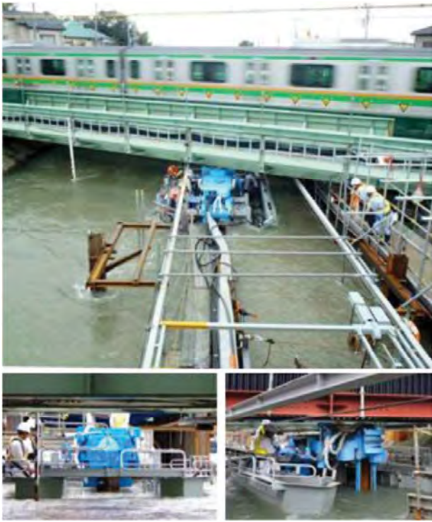
Figure 2. Press-in piling under a restriction of headroom (IPA, 2015).
