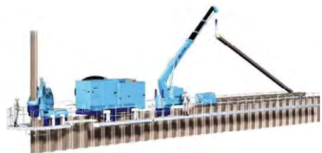
Figure 1. Press-in piling system saving temporary works (JPA, 2017).
