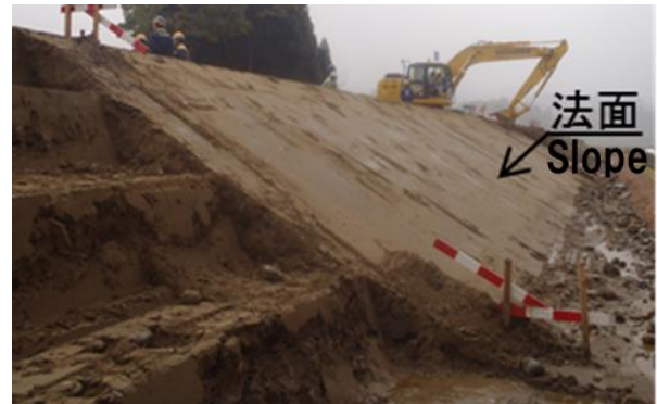
Fig. 15 Slope construction by Hydraulic excavator
