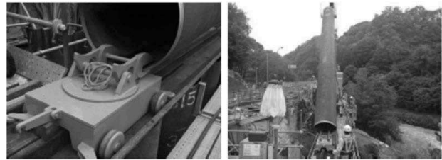
Figure 15. Lifting a tubular pile with a Pile Roller.
