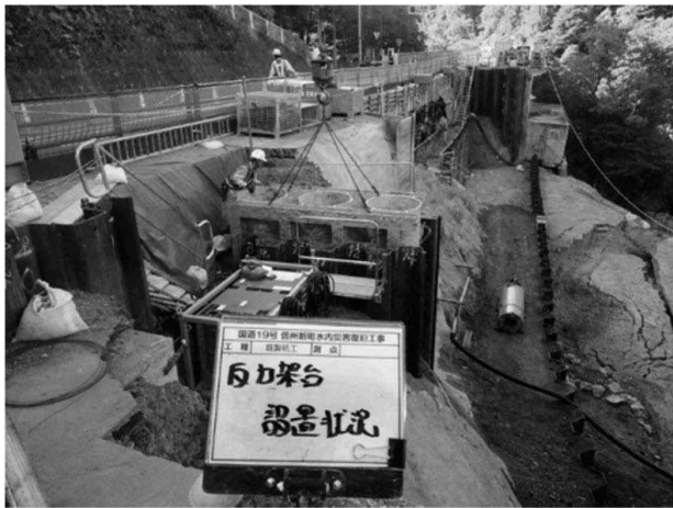
Figure 10. Installation of a Reaction Stand for tubular piles.
