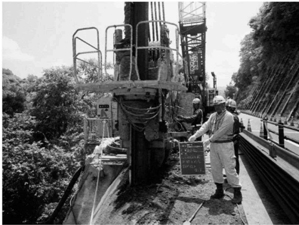
Figure 9. Installation of reaction piles.
