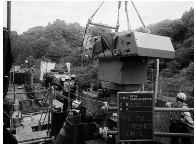
Figure 12. Assembly of a clamping crane.
