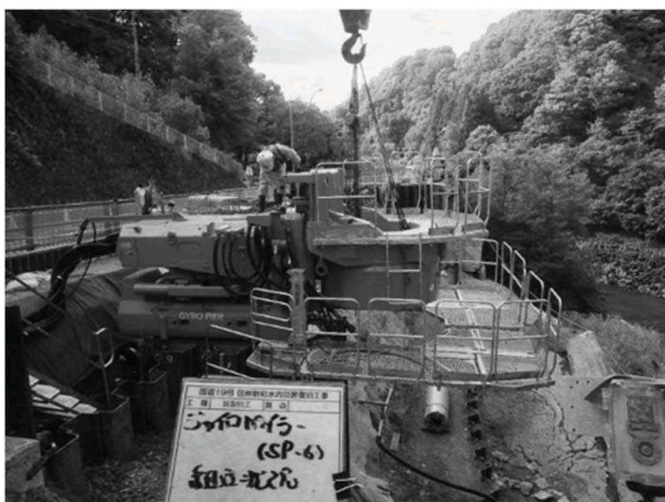
Figure 11. Assembly of a Gyro Piler.
