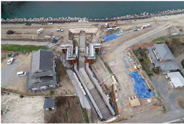
Photo 12. Successive construction work for the sluiceway.
