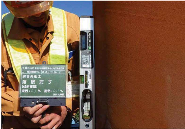
Photo 6. Measurement of verticality.
