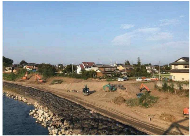
Photo 1. Preparing construction yard.
