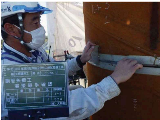
Photo 7. Checking root length and misalignment.
