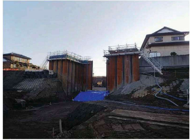
Photo 10. Completion of the construction of the pile wall.
