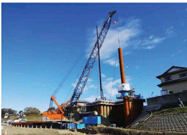
Photo 8. Verticality and centricity were surveyed during the piling procedure.
