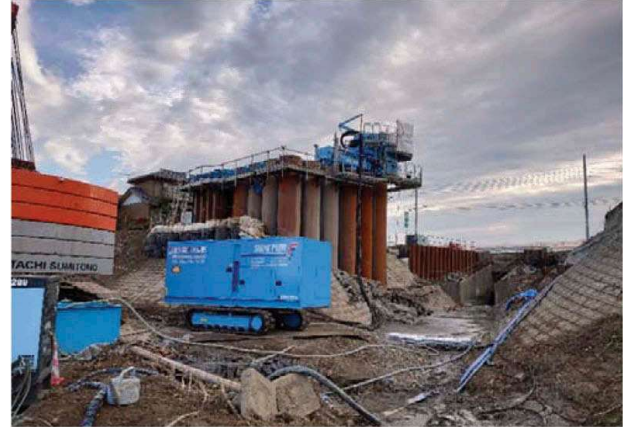
Photo 9. Piling work at high place.
