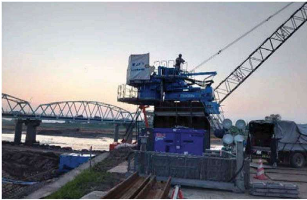
Photo 2. Reaction base supported by reaction sheet piles.
