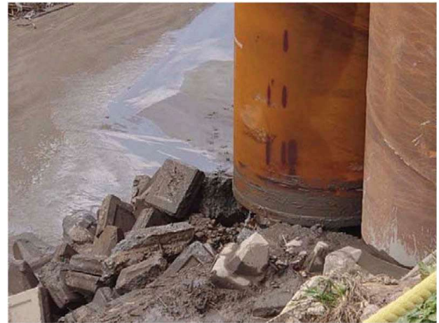
Photo 4. Concrete blocks cut and removed.
