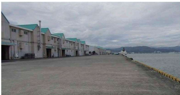
Figure 2. Existing buildings and a quay.
