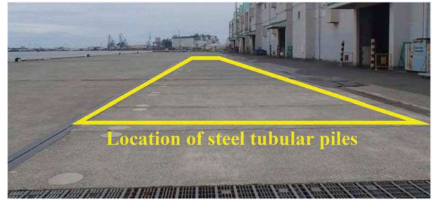
Figure 5. Working Yard before removal of pavement for the installation.
