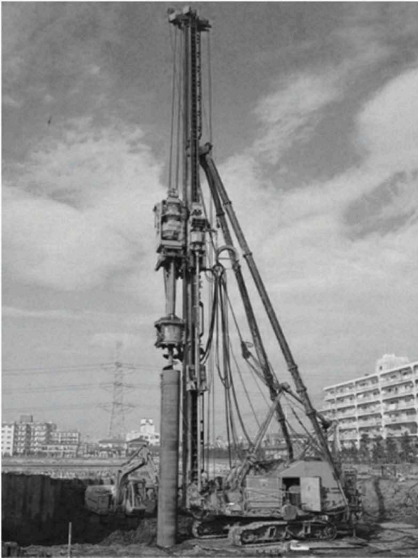
Figure 4. Leader rig mounted press-in system assisted by augering (Yamashita et al. 2010).
