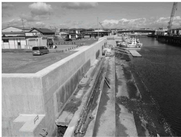
Figure 26. Newly constructed breast wall as seawall (South Side).
