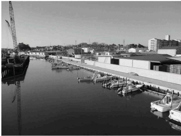
Figure 25. Newly constructed breast wall as seawall (North side).
