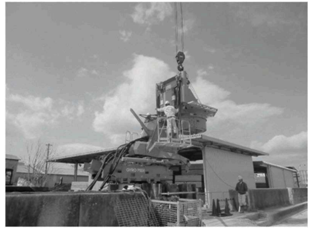
Figure 15. Assembly of Gyro Piler.
