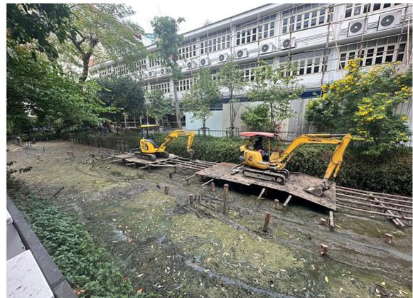
**Fig. 4** Timber platform and small excavator
