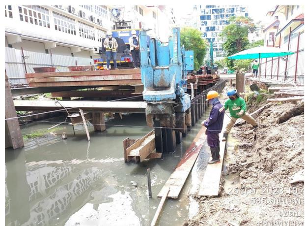
Fig. 16 Alignment of sheet pile pressing-in
