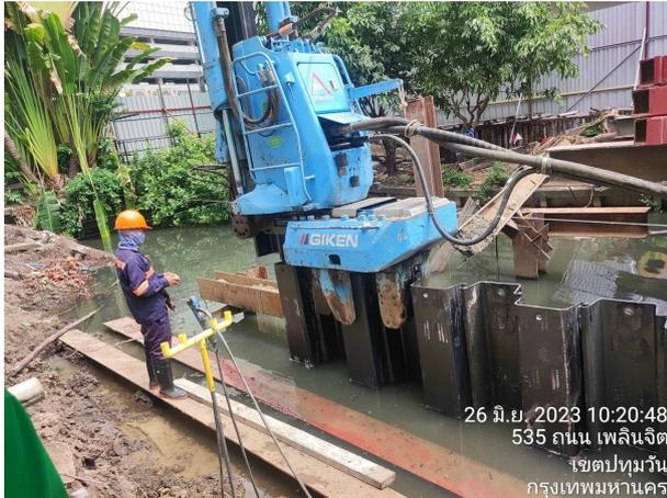
Fig. 17 SILENT PILER driving forward
