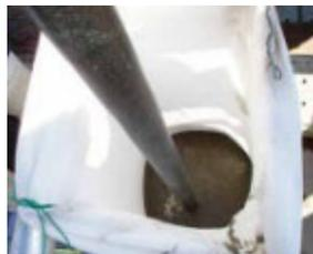
Fig.18 Mortar filling
