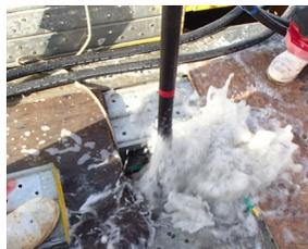
Fig.17 Washing between piles
