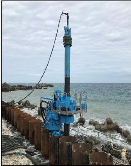
Fig.13 Installation of closure pipes in progress
