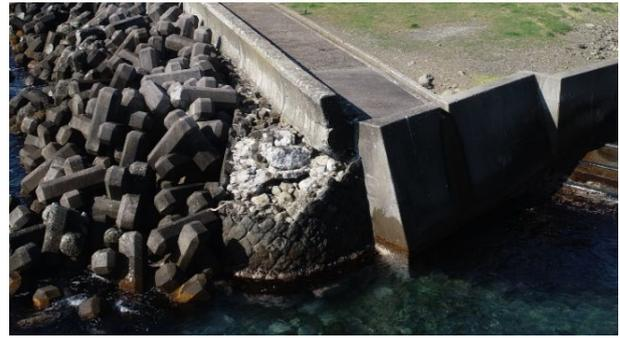
Fig.2 Collapse of coastal seawall
