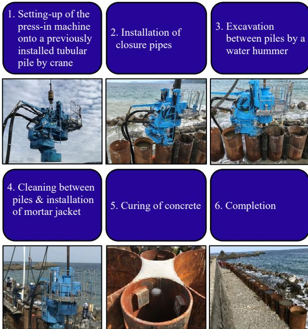
Fig.16 Sequence of waterproofing works
