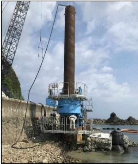
Fig.7 Installation of tubular piles by the Gyropress Method™
