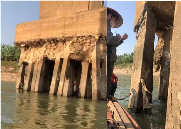
Fig. 1 The damaged Trung Ha bridge in Vietnam in 2023.
