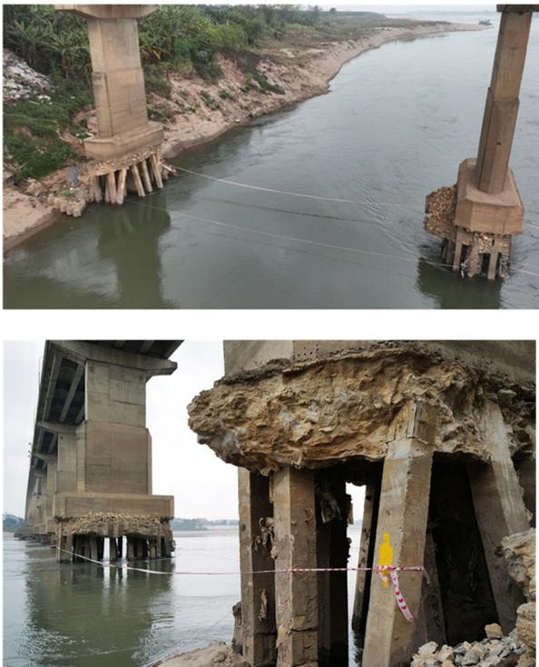
**Fig. 10** Damaged bridges need reinforcement.
