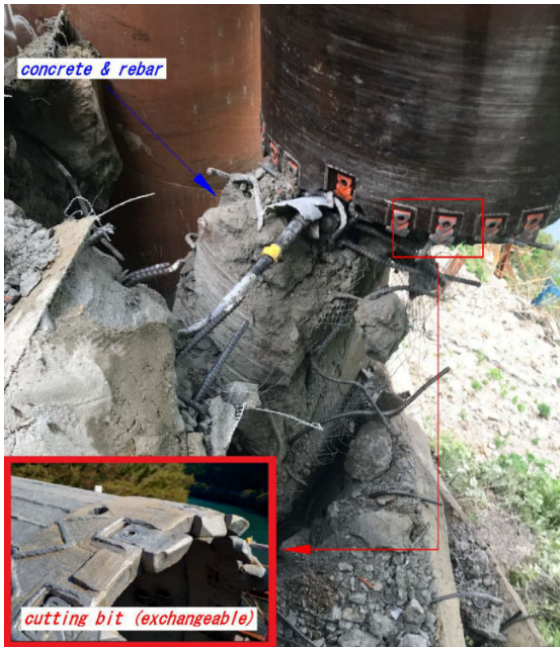
Figure 12. Removing work by core barrel
