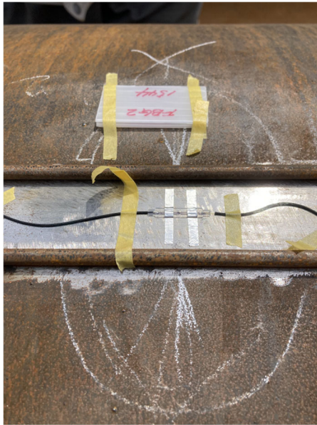
(a) Installation of FBG
