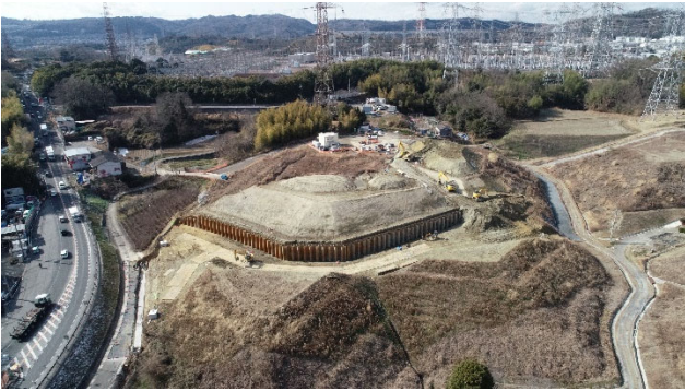
Fig. 11 Completion of Combi-gyro wall
