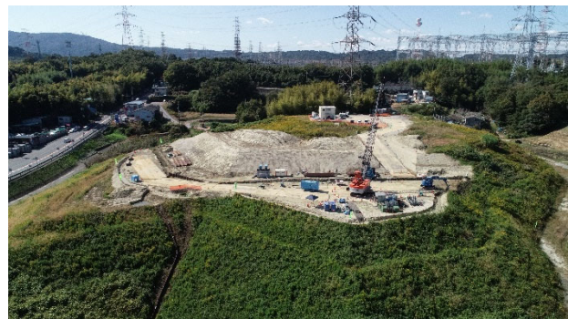
Fig. 9 Overview of the construction site
