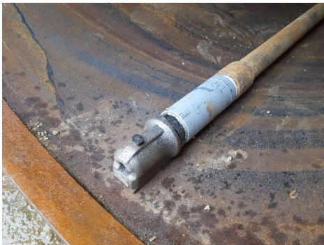
Fig. 6 Water jet pipe installed inside the tubular pile
