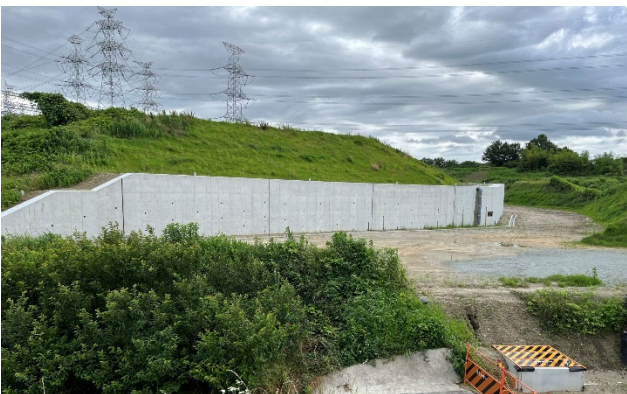
Fig. 13 Completion of the architectural concrete wall
