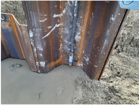
Fig. 5 Press-in with water jetting for Hat pile
