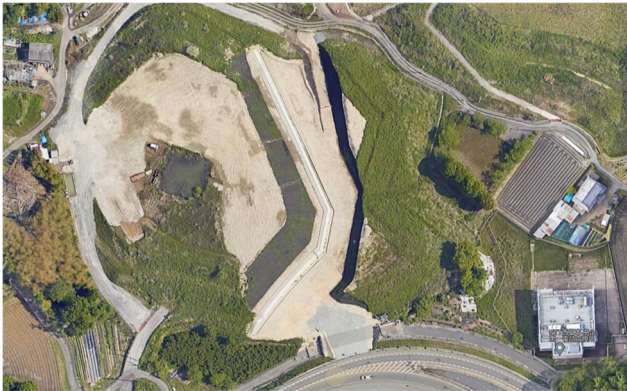
Fig. 12 Completion of the architectural concrete wall
