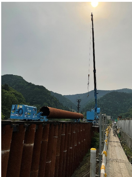
Fig. 12 Pile conveyed by Pile Runner
