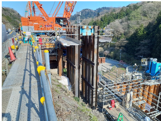
Fig. 5 Reaction frame set on the H-shaped beams
