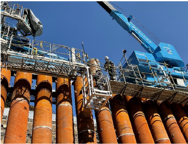
Fig. 6 The stage modified for welding work
