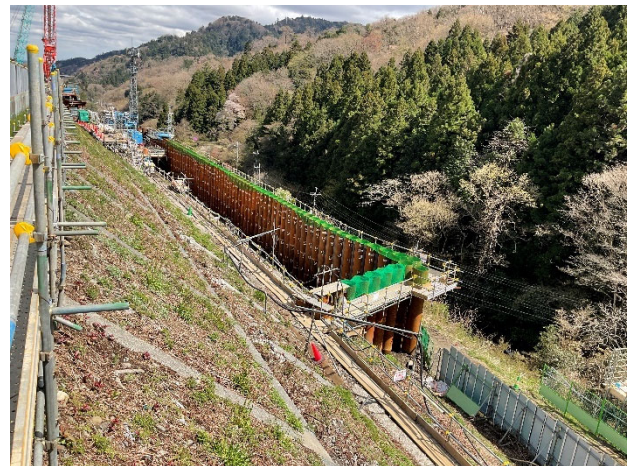
Fig. 14 Completion of piling of B-Line
