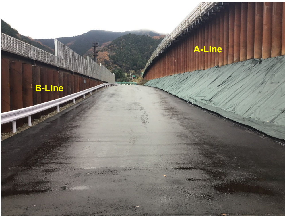
Fig. 15 Completion of access road
