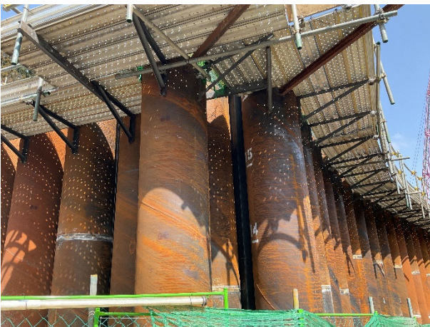
Fig. 7 Looking up at the work passage
