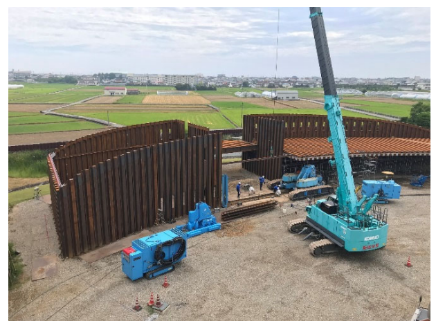
Fig. 30 The Press-in machine on the Reaction Stand with crawler unit
