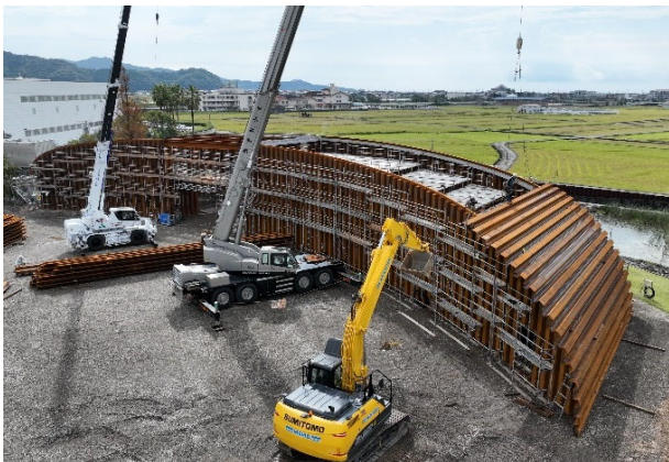
Fig. 32 Roof sheet pile installation
