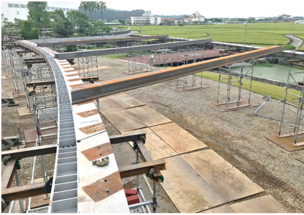
Fig. 25 Second floor connecting beam installation
