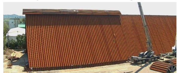
Fig. 22 Circular roof installation
