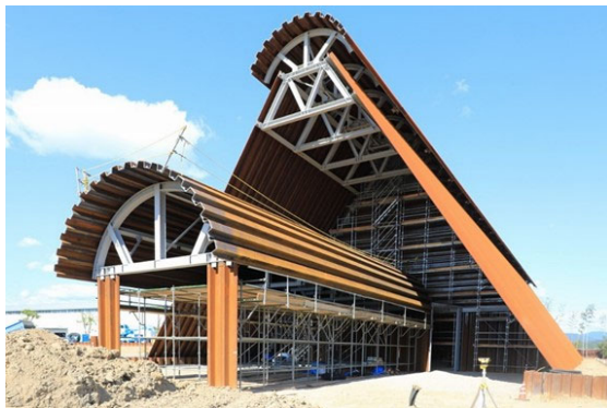
Fig. 24 Porch section construction
