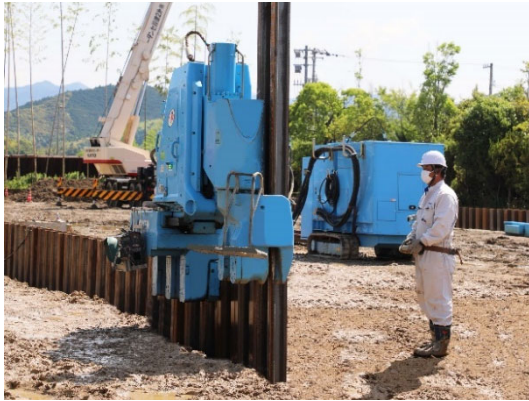
Fig. 17 Press-in of steel sheet pile
