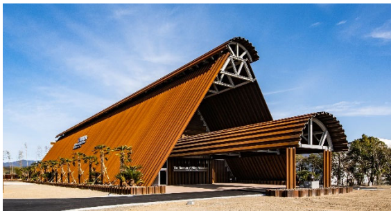
Fig. 26 Photo of completion
