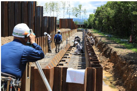
Fig. 18 Installation of column legs (steel foundation)
