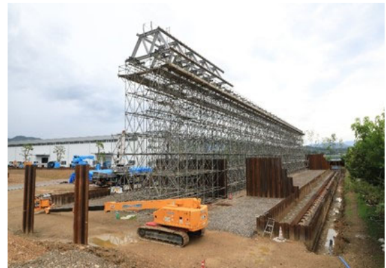
Fig. 19 Support scaffold assembly and trapezoidal frame installation
