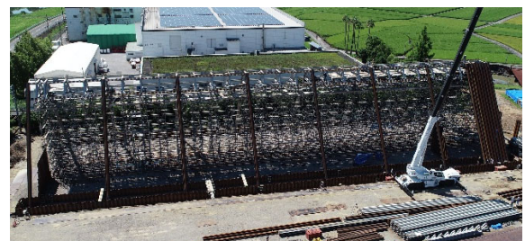
Fig. 20 Steel sheet pile construction on both sides of diagonal wall
