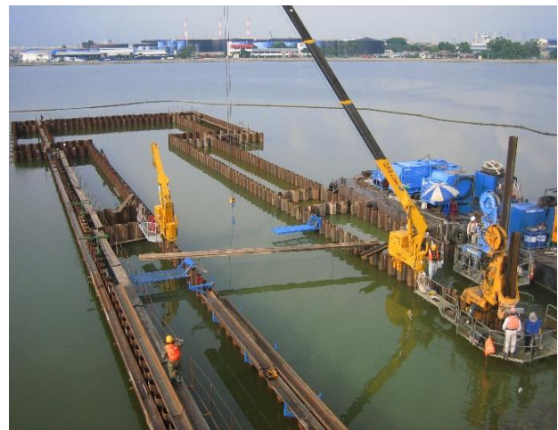
Fig. 6 Non-staging press-in piling (GRB System)
