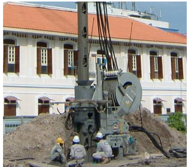
Fig. 3 Sheet piles installed by Super Crush System
