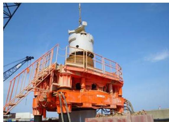
Photo 1. Overview of Pipe drill
