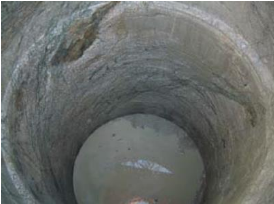
Photo 7. Drilled wall after excavation
