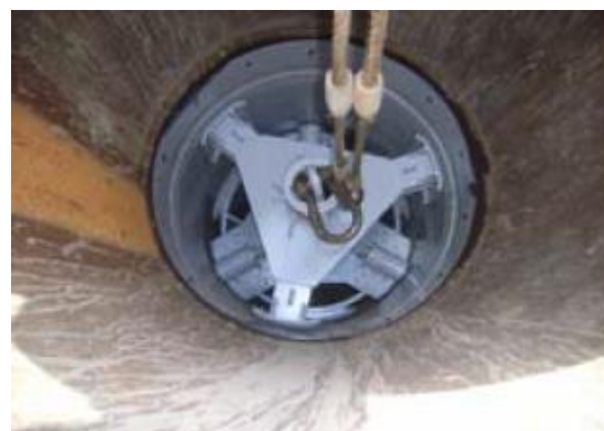
Photo 6. Pipe drill setting status
