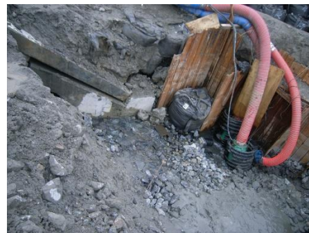
Fig. 16 Drainage pump to lower the water level inside the sheet piles
