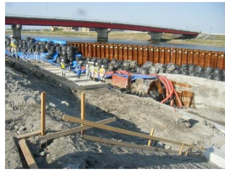
Fig. 15 Additional measure to prevent the sheet pile deformation with sandbags
