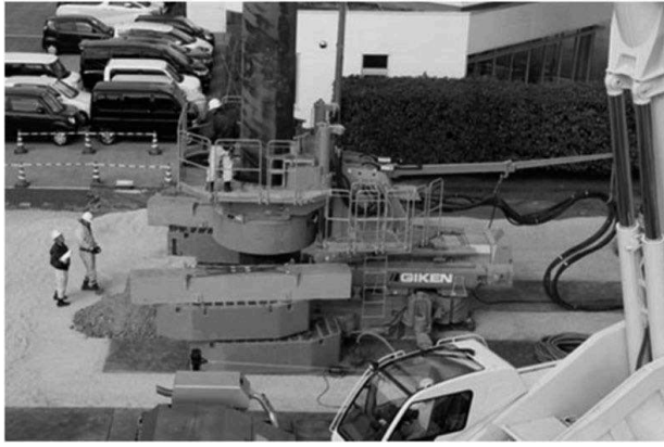
Figure 3. Press-in machine with Self-weight system.
