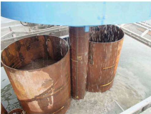
Figure 11 . Closure pile installation.
