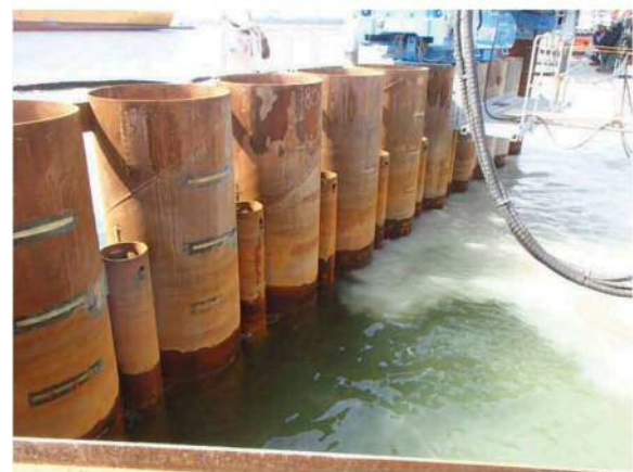
(c) Piles Installation Process
