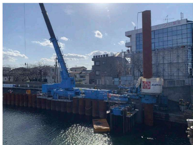
Figure 8. Piling state during Step 8 and 9.
