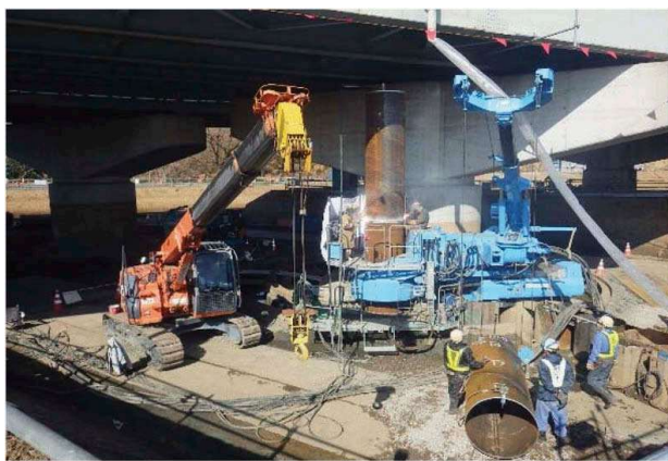
Figure 14. Piling work beneath a girder.
