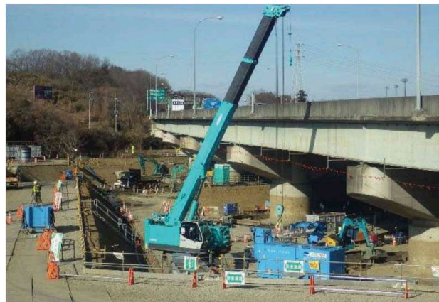
Figure 13. Piling work at the open place.
