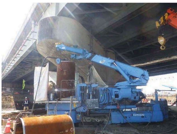
Figure 9. Hoisting system for low headroom in operation.
