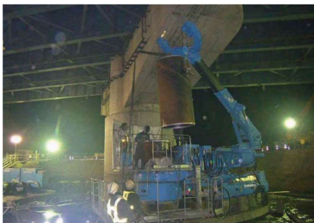
Figure 3. Piling at night.
