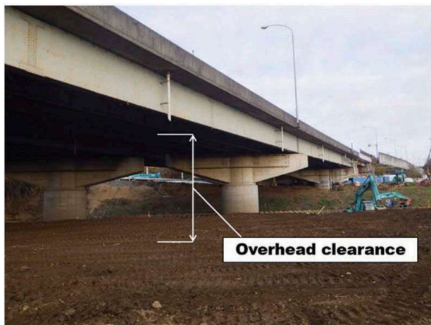
Figure 2. Overhead clearance under the Oppe River Bridge.
