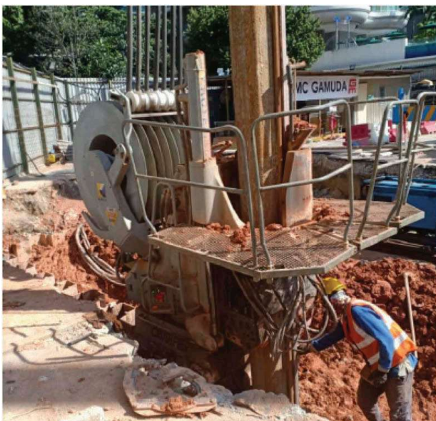
Figure 15. Super crush piler are working on site (Yun, 2020).
