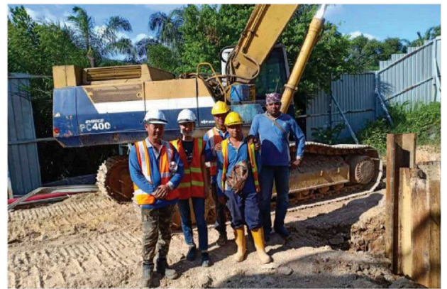
Figure 13. Student spending their time at the actual construction site (Yun, 2020).
