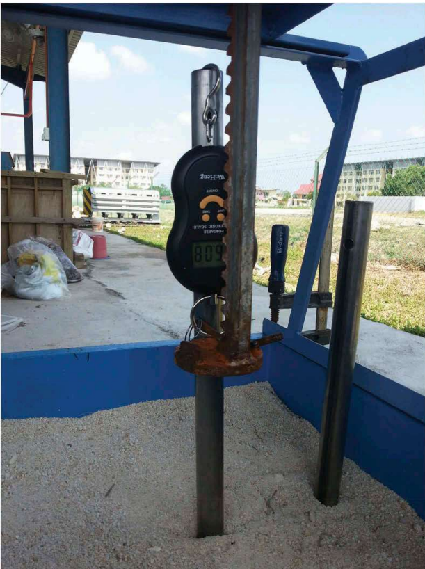
Figure 23. Pile installation force monitoring setup.
