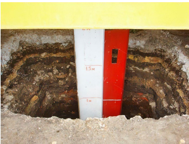
Figure 2. Driving and extracting the mobile pile element (on the right) through the interlock of the basic pile element (left)
