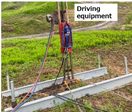
Fig. 9 A driving equipment for the installation of anchors
