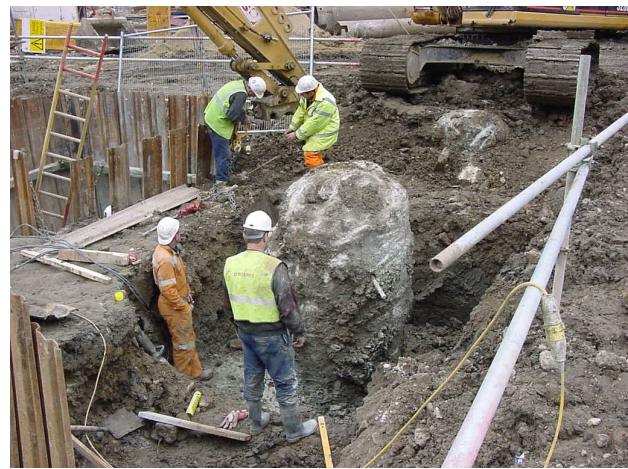
Figure 1 Typical large diameter pile on a redevelopment site
