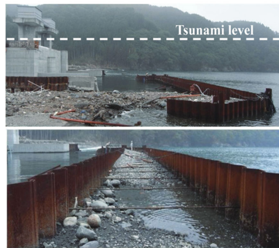
Fig. 2. The resilience of the double-sheet pile cofferdam following the impact of a 9-meter tsunami in Japan's Iwate Prefecture in 2011 (Otsushi et al., 2016).
