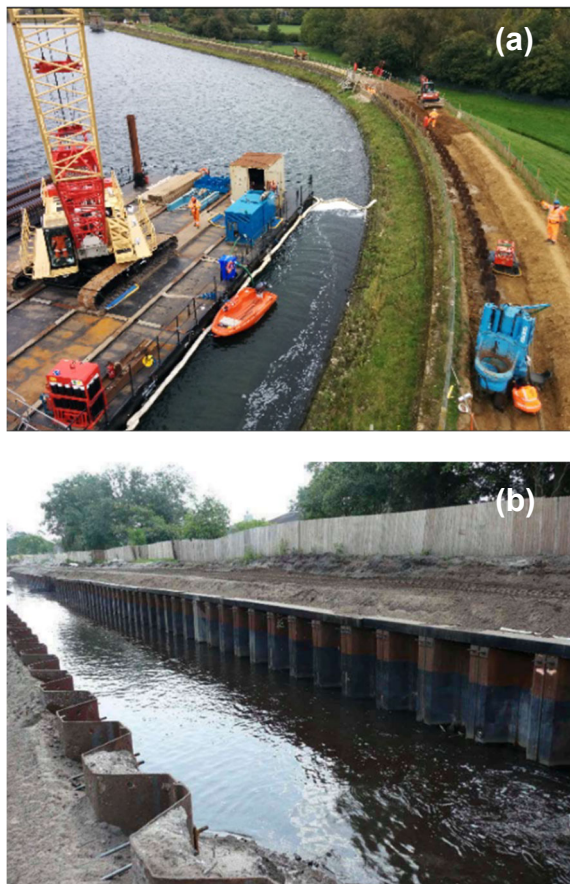
Fig. 5. (a) Example of installation of cut-off sheet pile walls by the GIKEN press-in pile machine (Island Barn Reservoir, United Kingdom) (b) Example of repair and upgrade of riverine levees by 950 pairs of sheet piles (USA).
