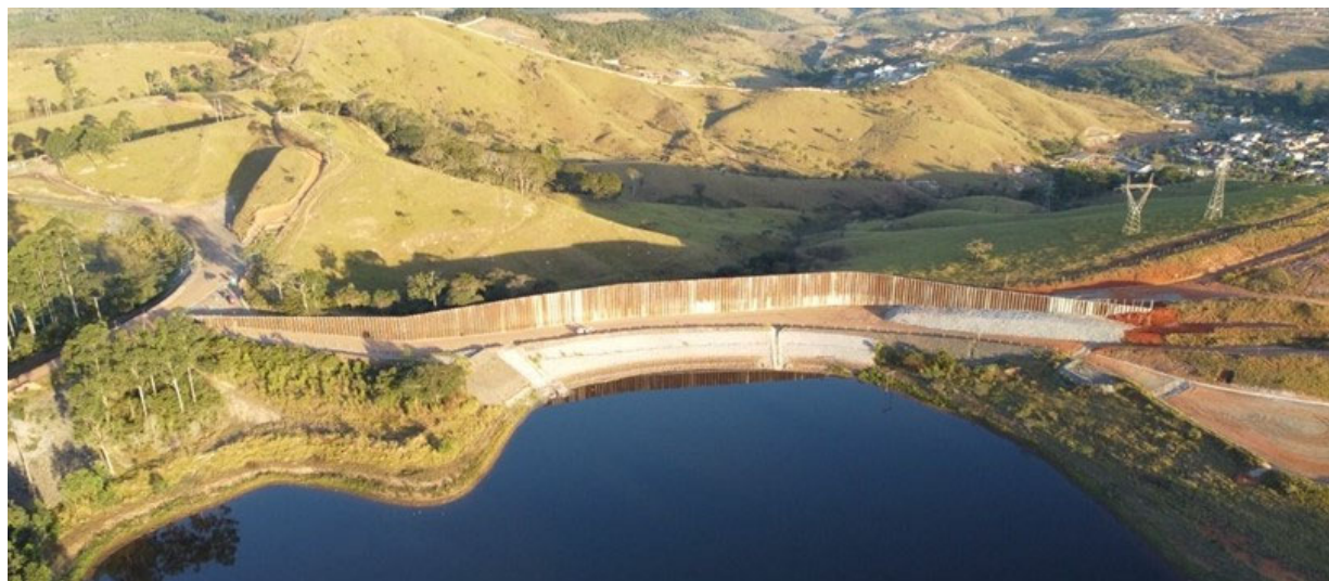
Figure. 20 Photograph of the piling operation
