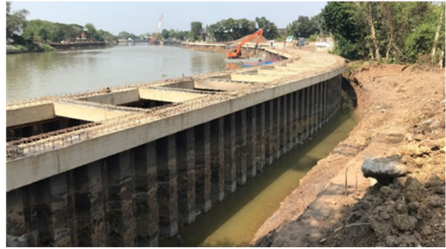
Figure 11. Filling soil between hat-type sheet piles
