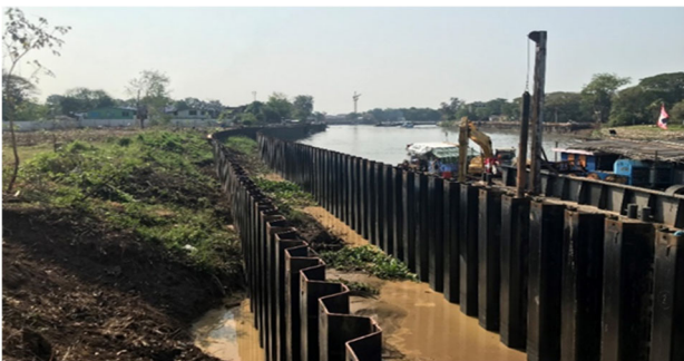
Figure 9. Double hat-type sheet pile wall
