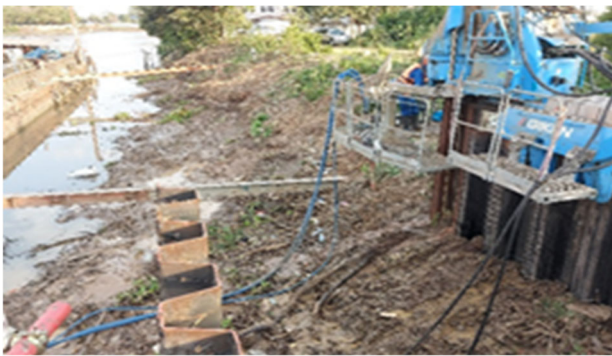
Figure 8. Press-in work
