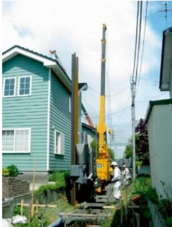
Fig.1 Example of installation of Zero Sheet Piles. (<https://www.giken.com/ja/solution/zero/>)
