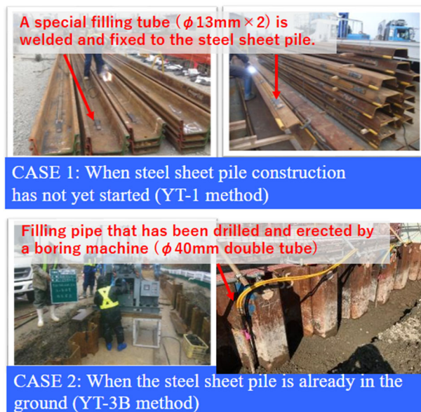
Fig.14 Installation type of filling pipe
