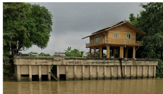
Fig. 4 Conventional type of riverbank protection wall
