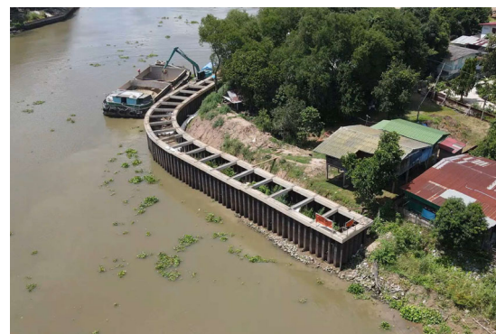
Fig. 10 Aerial view of nearly completed structures
