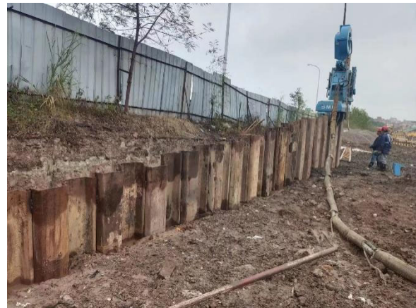
Fig. 3 Flood Prevention and Disaster Mitigation Emergency Projects - Standard Press-in
