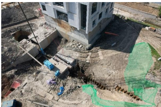
Fig. 7 Permanent Reinforcement Projects for River Embankments - Press-in with Water Jetting
