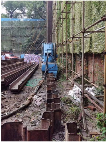
Fig. 5 Historical Building Renovation Projects - Standard Press-in
