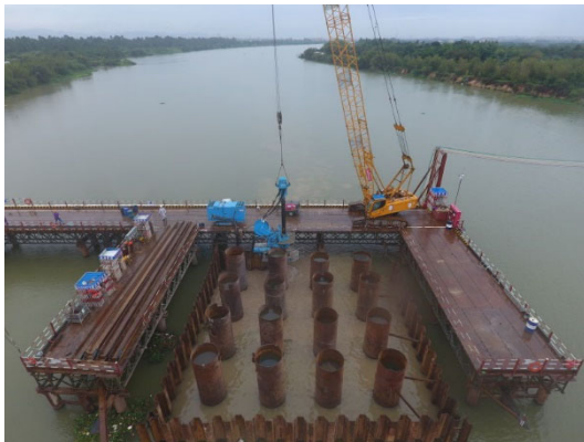
Fig. 6 Bridge Cofferdam Projects – Press-in with Integral Augering
