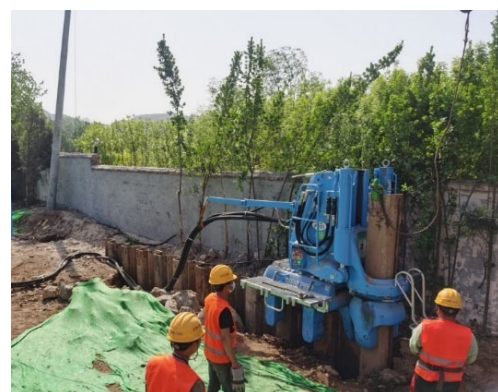
Fig. 4 Water Supply Pipeline Reconstruction Projects - Press-in with Water Jetting
