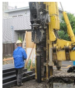
Fig. 2 Press-in pile driver
