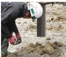
Fig. 1 Pile Tip of Kakuske-pile
