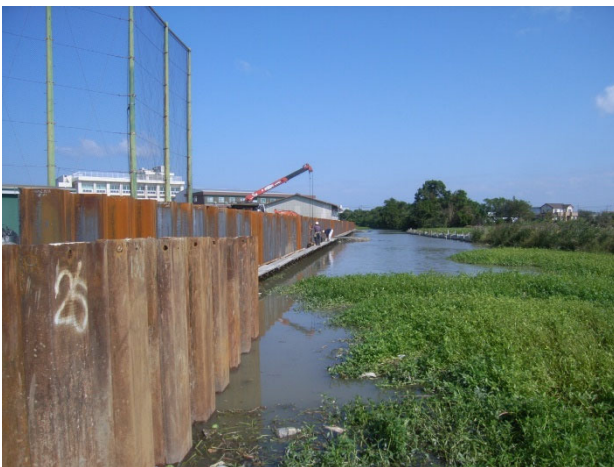
Fig. 12 Sheet pile wall installed along a waterway
