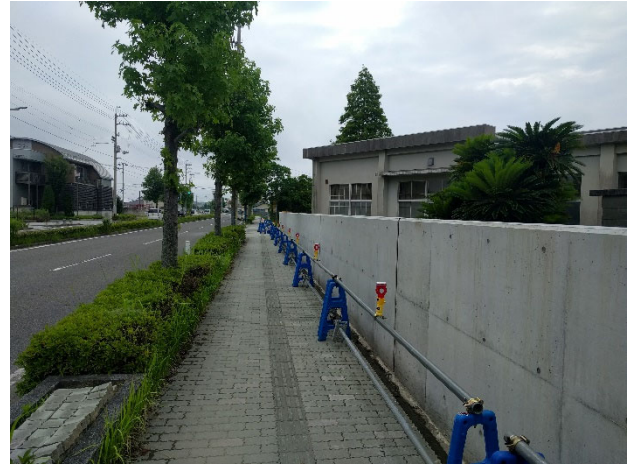
Fig. 13 Flood wall complete with concrete cover
