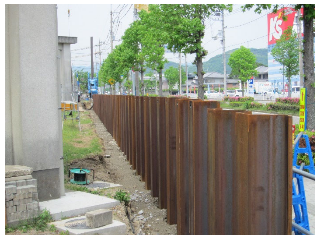
Fig. 10 Sheet piles installed next to school buildings with minimal clearance
