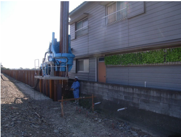
Fig. 11 Press-in sheet pile installation next to a house
