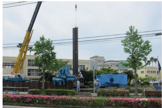
Fig. 9 Sheet pile installation in front of the high school's main entrance
