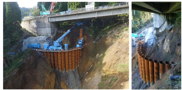
Fig. 19 Installation of tubular piles
