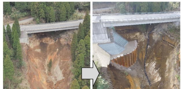
Fig. 20 Comparison of before and post construction
