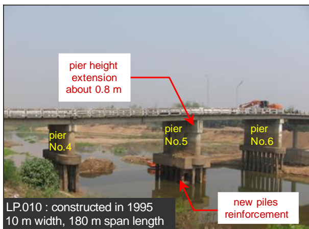
Fig. 3 Repair of the settled bridge LP.010 in Lamphun, Thailand (2008)
