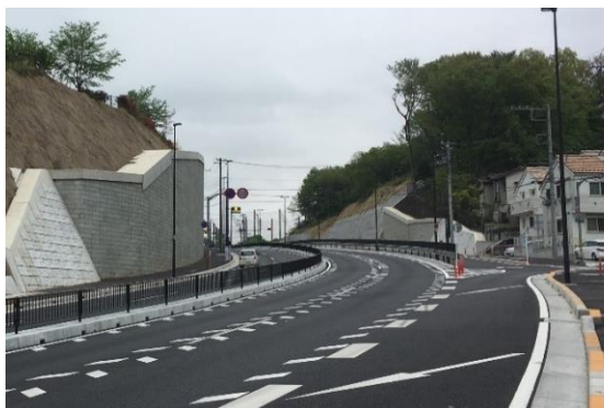
Fig. 8 Photo taken after construction
