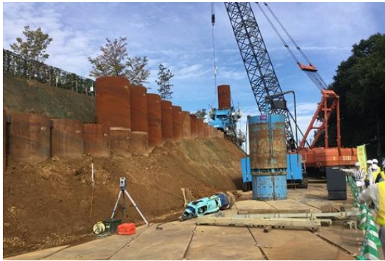
Fig. 7 Photo taken during construction
