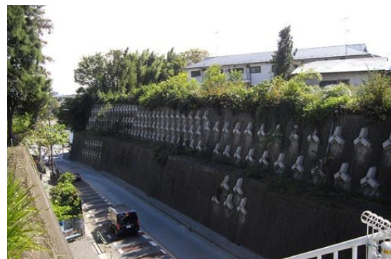
Fig. 2 Photo taken prior to construction
