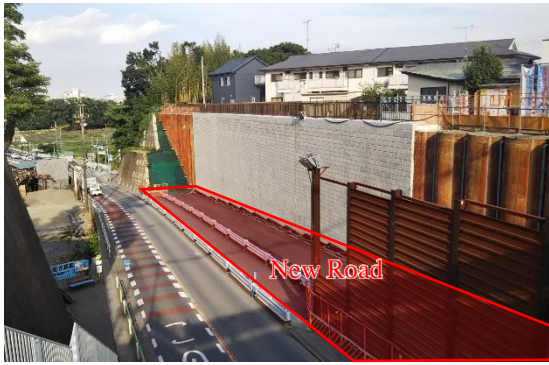
Fig. 4 Photo taken during construction of cladding panels
