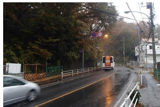
Fig. 6 Photo taken prior to construction
