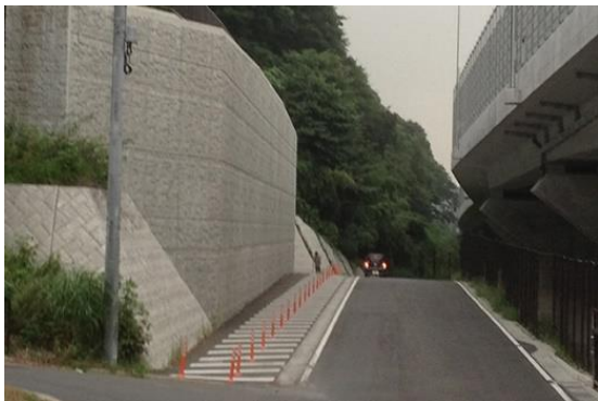
Fig. 11 Photo taken after construction
