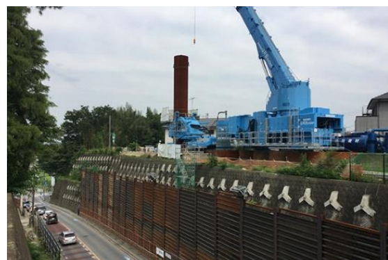
Fig. 3 Photo taken during pressing-in steel tubular pile
