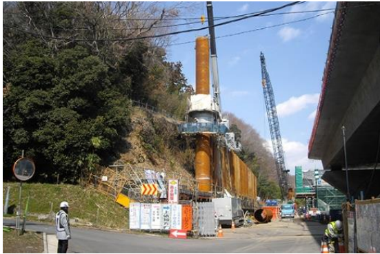
Fig. 10 Photo taken during construction
