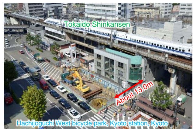
Fig. 22 Excavation of inner soil (construction status)
