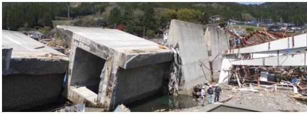
(a) Gravity-type levee.
