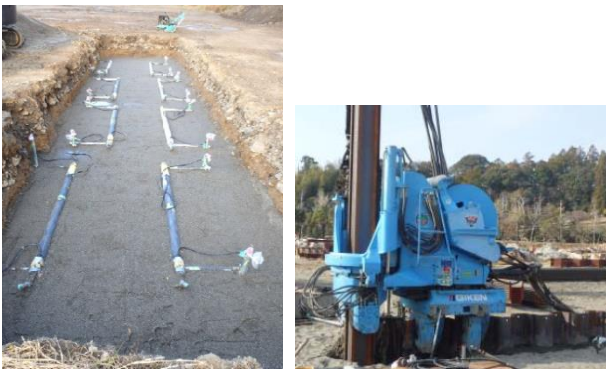
Fig. 2 State of gas pipes and press-in construction
