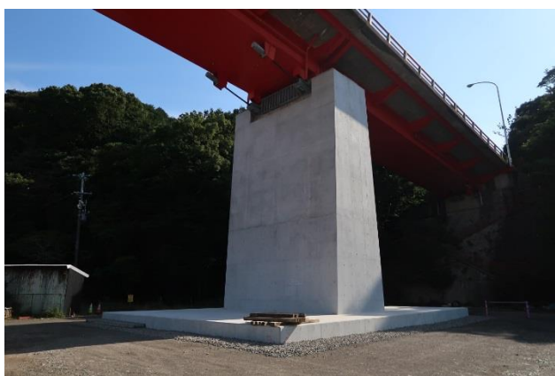
Photo 6. Completion of the aseismic reinforcement work
