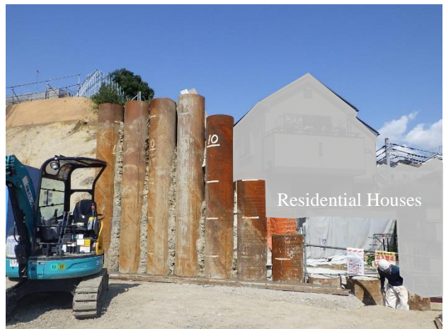
Fig. 7 Cut steel tubular piles after the excavation
