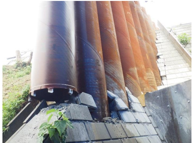
Photo 1. Installation of steel tubular piles directly into concrete retaining wall
