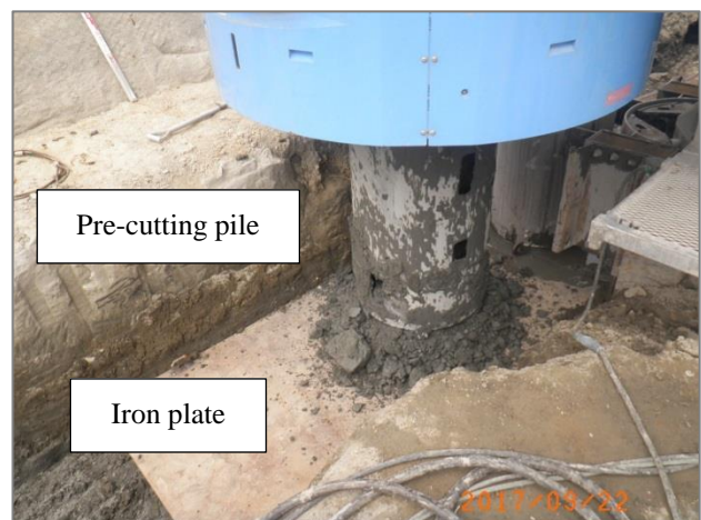
Photo 3. Pre-cutting pile
