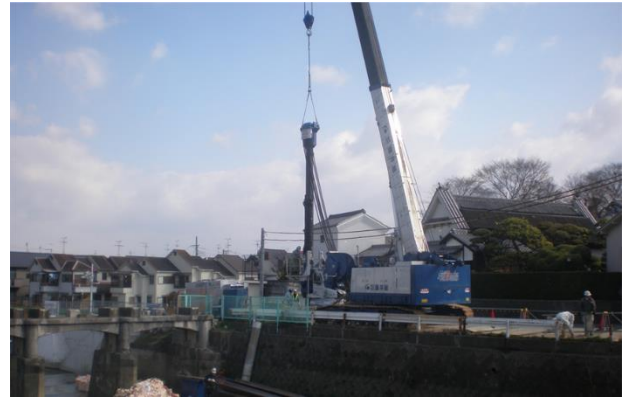
Photo 2. Construction site (during construction)
