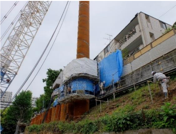
Photo 6. Construction adjacent to the existing building
