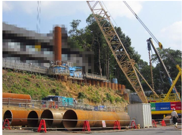
Photo 4. Construction adjacent to the existing building
