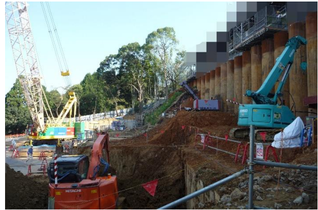
Photo 3. Photo taken at the construction site
