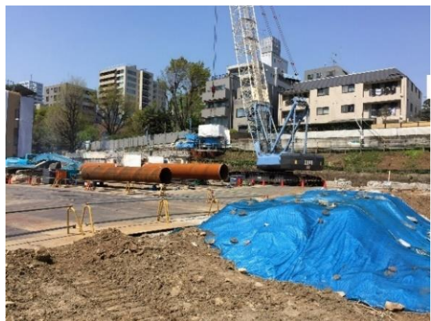
Photo 5. Photo taken at the construction site
