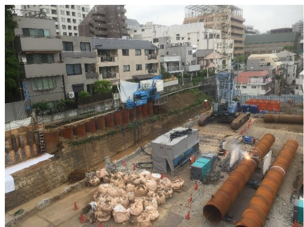
Photo 1. Construction of earth retaining wall in urban area
