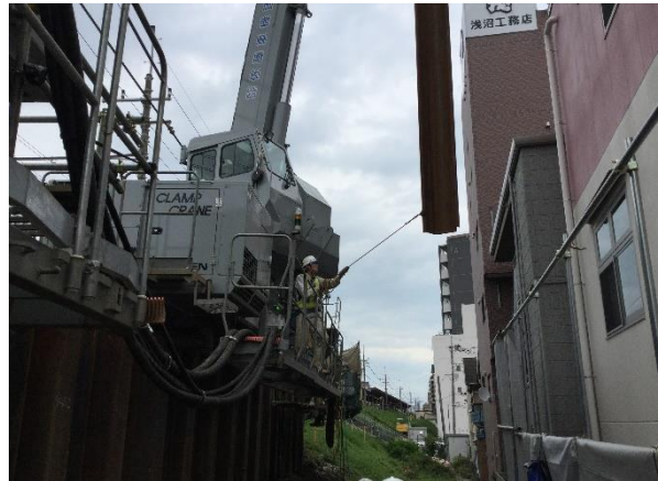
Photo 6. Clamp crane slewing at the minimum radius
