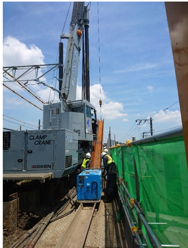
Photo 3. Pile conveyed underneath the clamp crane
