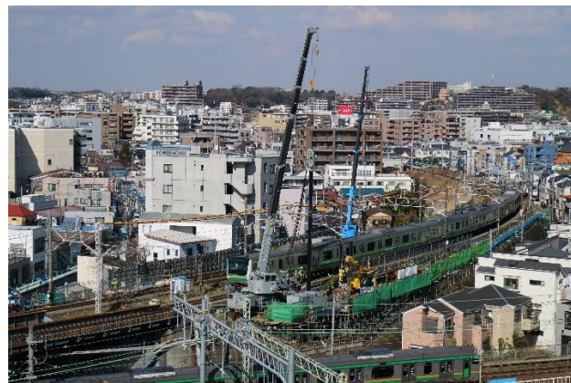
Photo 4. Two crush pilers with system conducting sheet piling on the both side of the embankment
